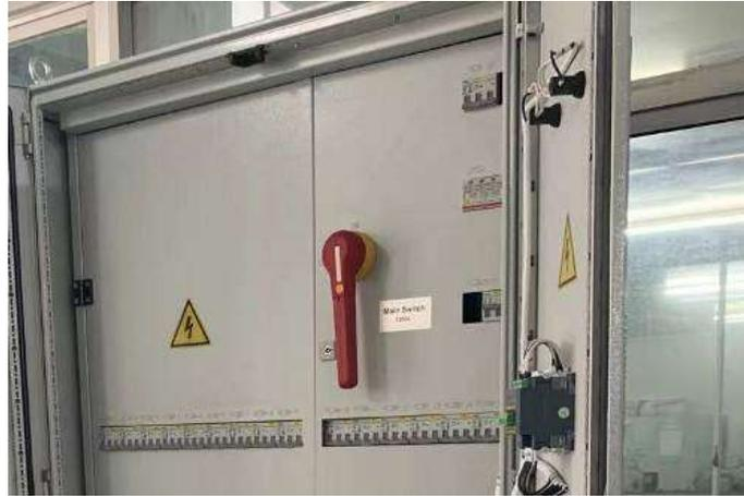
Figure 5-1-5 Schematic diagram of the main air switch of PDC
