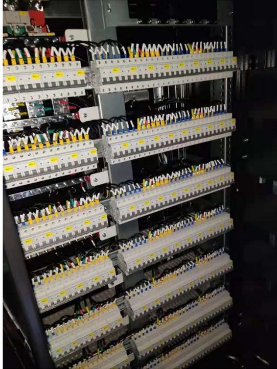
Figure 5-1-3 Schematic diagram of the air switch of a PDC
