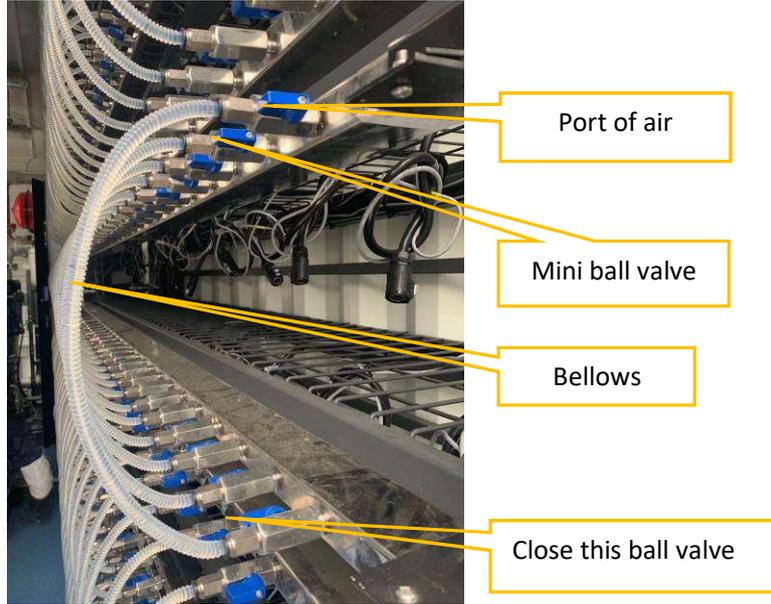
Figure 5-5 System - ball valve for connecting pipelines
