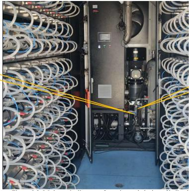
Status of closing: the handle of ball valve is perpendicular to the pipeline.
