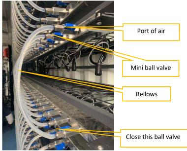
Figure 5-2-5 System - ball valve for connecting pipelines
