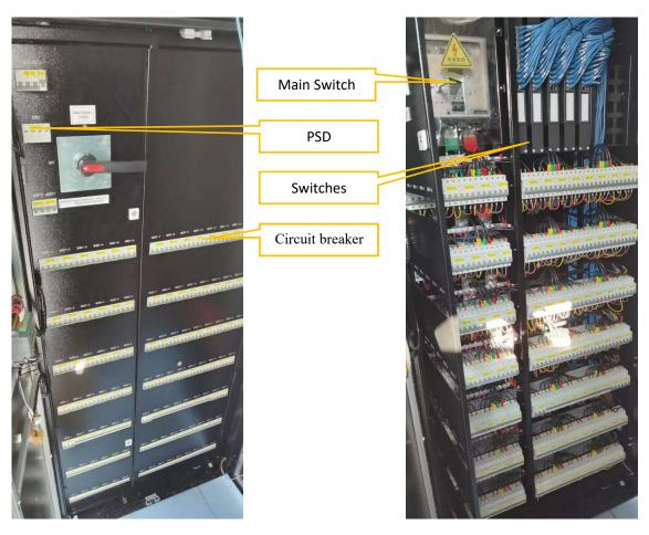
Figure 4-2-9 Internal view 01 of PDC
