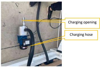
Figure 5-3-4 Pump station - charging hose
